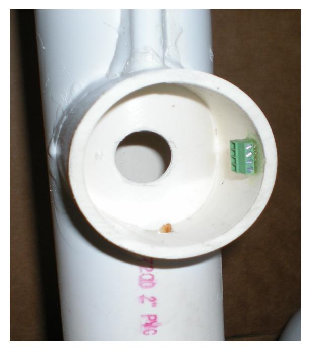
This view shows the cable hole in the bottom of the saddle, which also doubles to allow any water that might get in to weep out of the bottom of the junction box.
